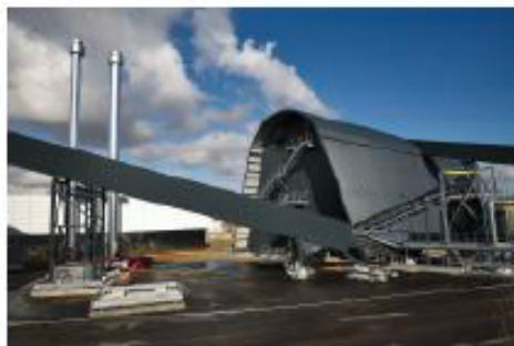
34 MW biomass heating facility in Lyon. https://www.usrenouvelable.com/
